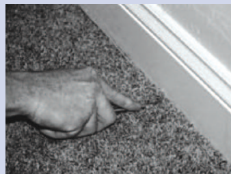
Figure 5. Stretching and tucking the loop wire along the baseboard.
