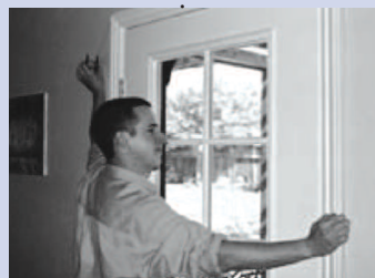
Figure 6. Pulling the loop wire taut around a doorway where there is no carpet.
